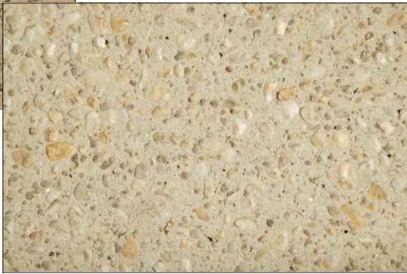
Combination of rock salt and exposed aggregate or grit blast concrete in earthy tones to areas around the Commons.
